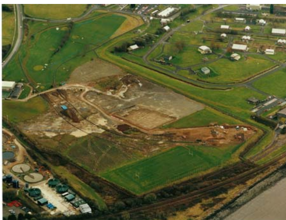
Drill Rig Site at Saltash
