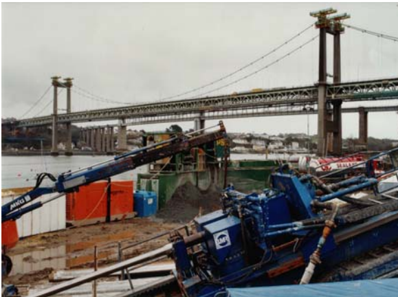
Drill Rig Site at Saltash
