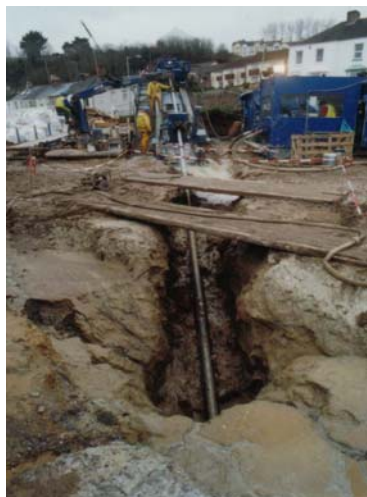
Rig Site at Saltash
