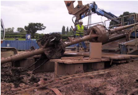
Hole Opener and Centraliser Hole Opening Complete
