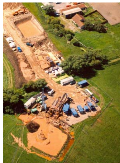
Kenn Moor Road Drill Site
