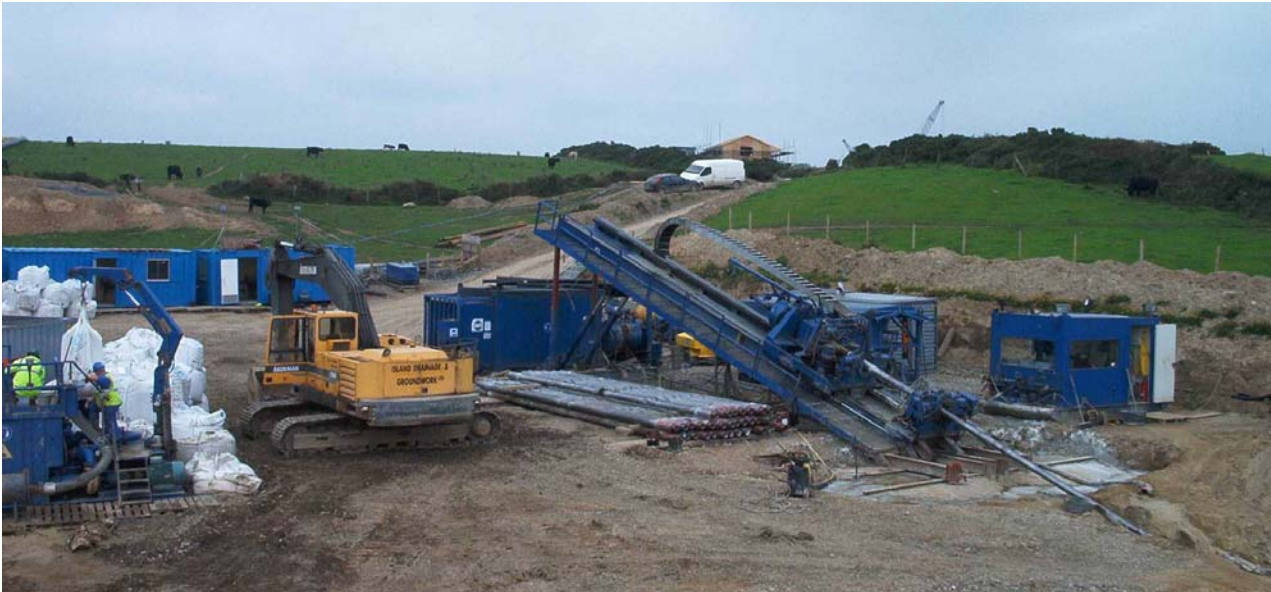
Drill Rig Site at Meary Veg
