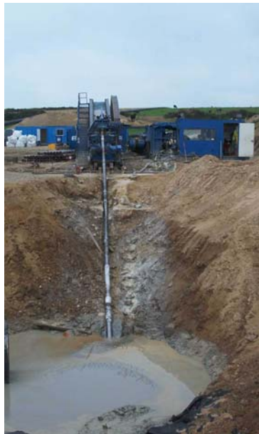
Pilot Drilling
