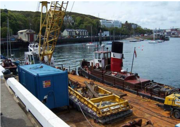
Concrete Mattresses Loaded for Placement over Pipe
