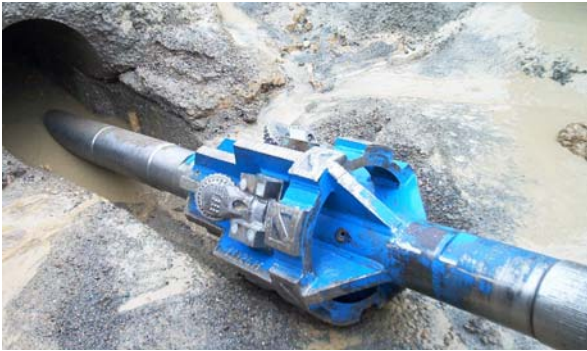
Hole Opener Commencing Run
