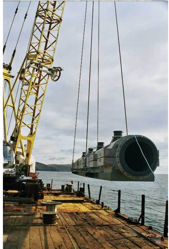
Lowering Diffuser to Seabed
