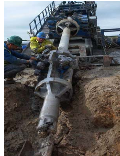
Hole Opener Assembly
