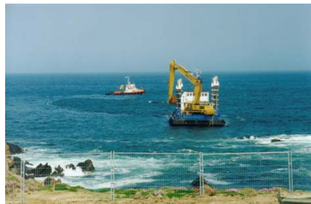
Marine Equipment Preparing for Pipe Pull
