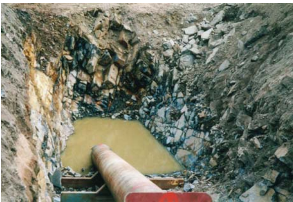
Installation of Casing Pipe
