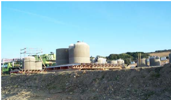
Casting of Concrete Diffuser Domes
