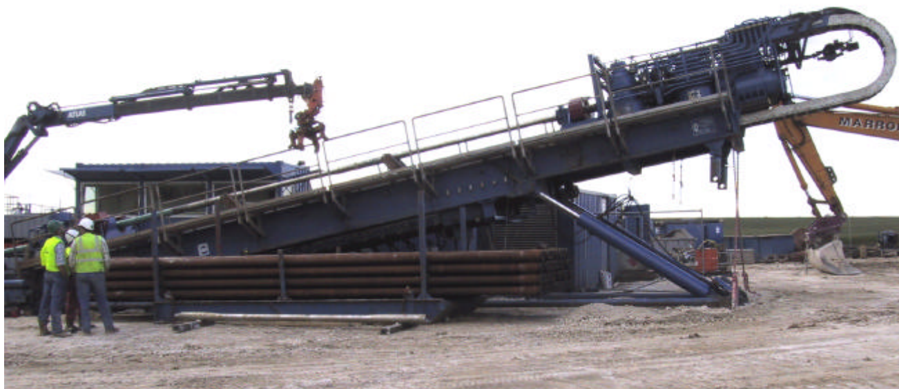
Fig. 1 LMR's 300 Ton Drilling Rig
