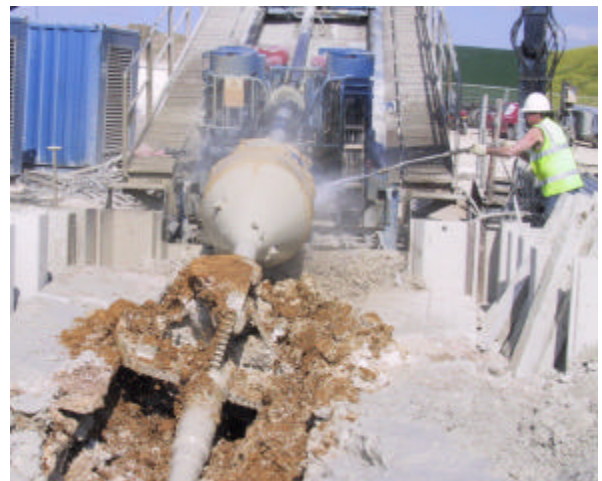
Fig. 3 The 58" Hole-Opener Coming Out of Hole
