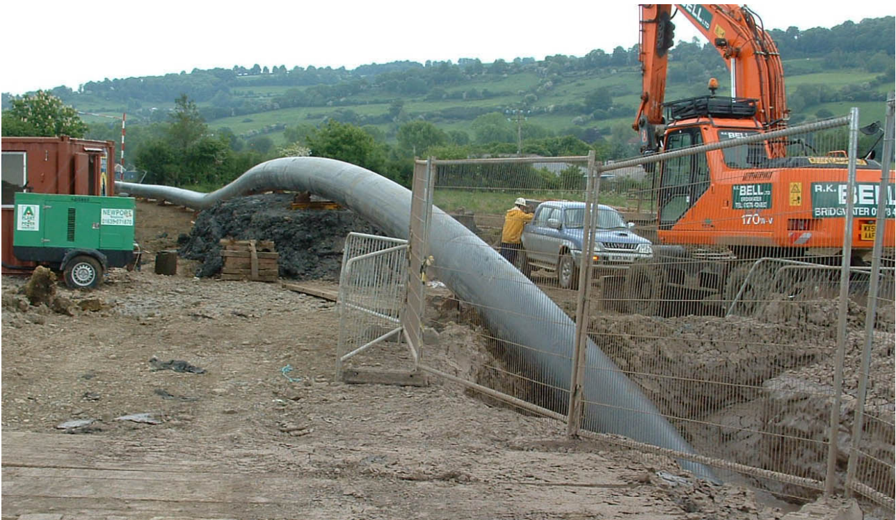
Fig. 6: Shows Product Pipe Overbend Construction
