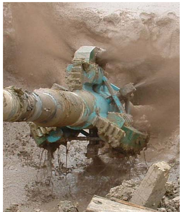
Fig. 3: The 40" Hole-Opener at the Start of the Pass
