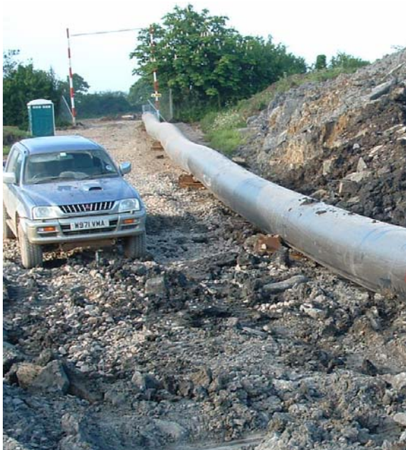
Fig. 4: The 800 mm Product Pipe on Rollers
