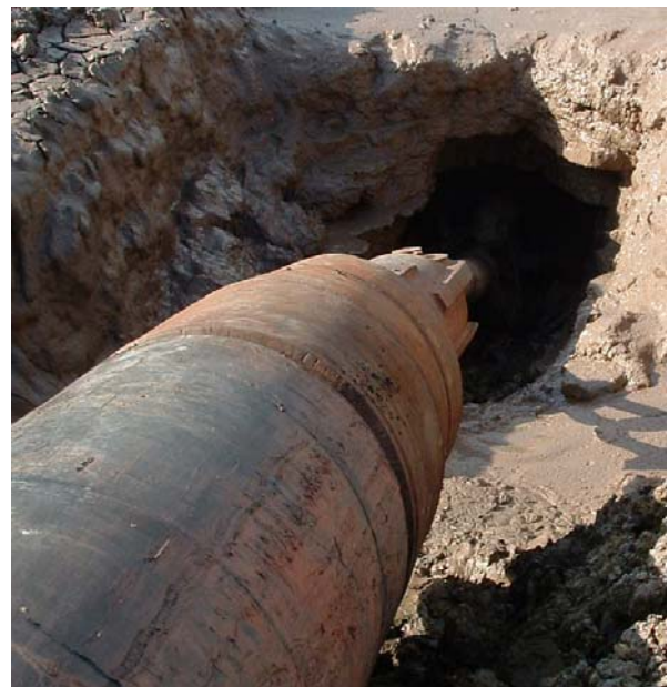
Fig. 5: Pulling Head Prior to Going into Hole During Pullback
